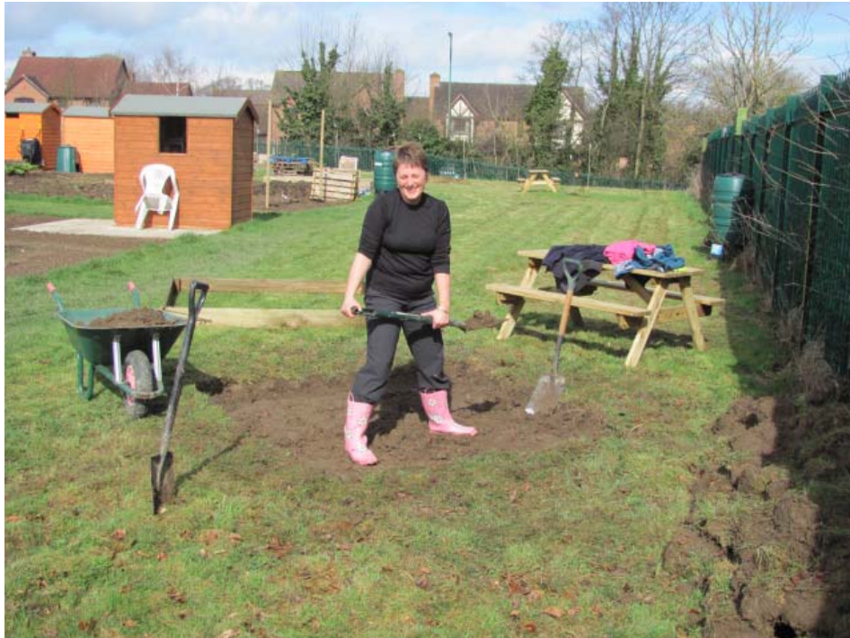
Digging out the base for one of the picnic benches.
